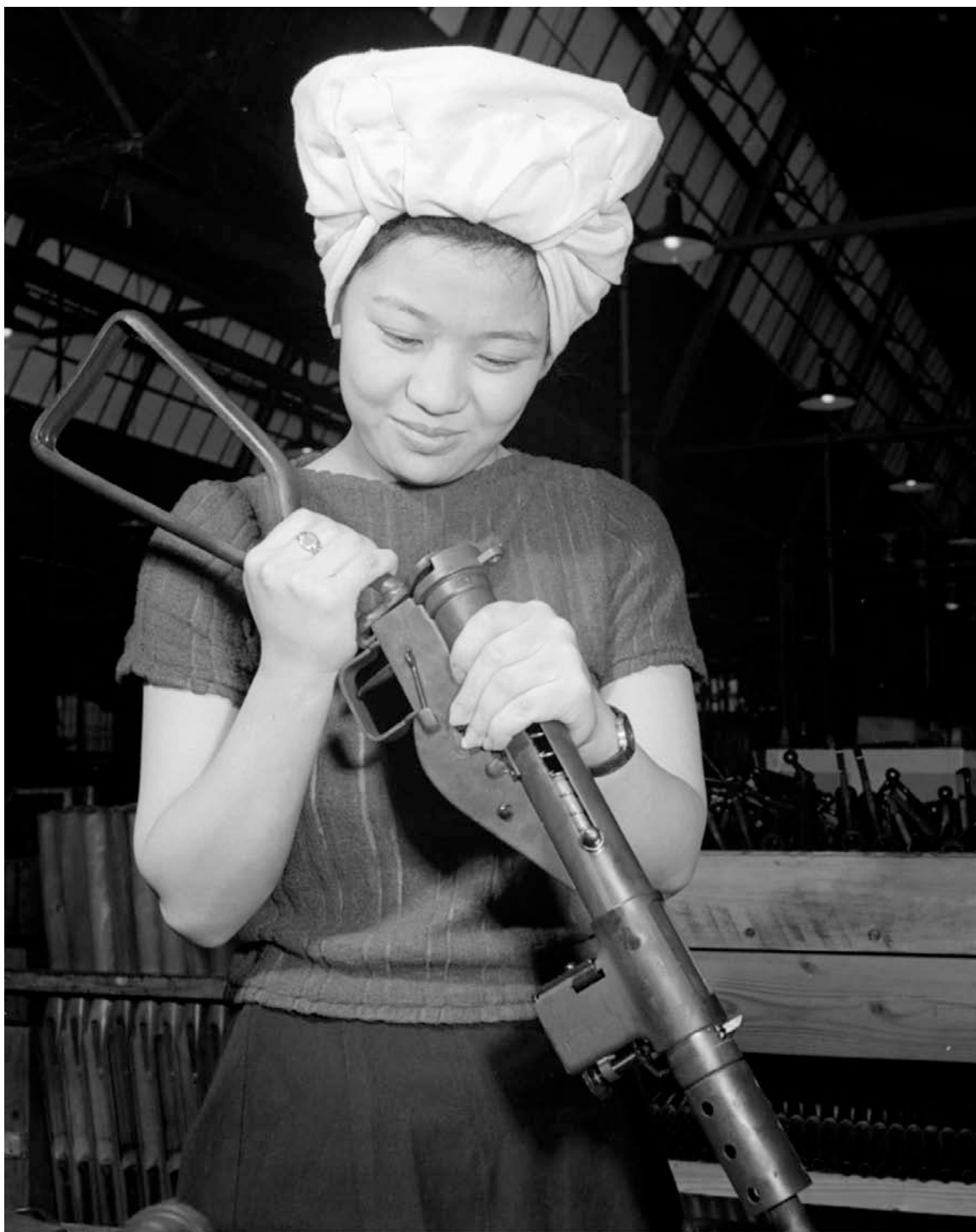
Title: Unidentified Chinese female munitions worker adding a butt to the end of a gun at the John Inglis Company plant Date: April 10, 1944 Source: Library and Archives Canada Identification number: e000762940
